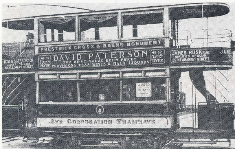
Car 23 or 24 in original condition. Note the route board and the bamboo pole carried below the rocker panel.
